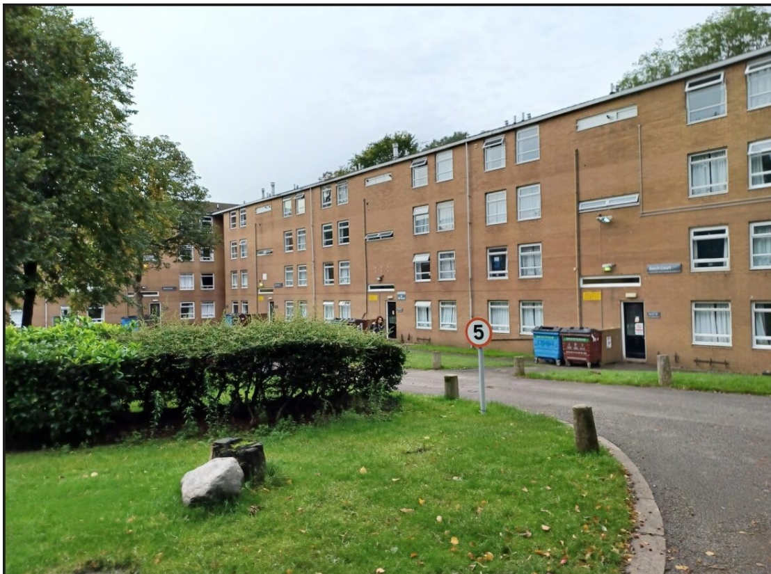
Existing Campus Building (Beech Court)
